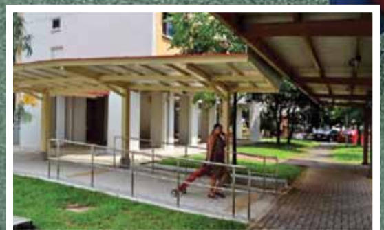
Covered linkway from existing linkway to Blk 432 Jurong West St 42 (Jurong Central)
