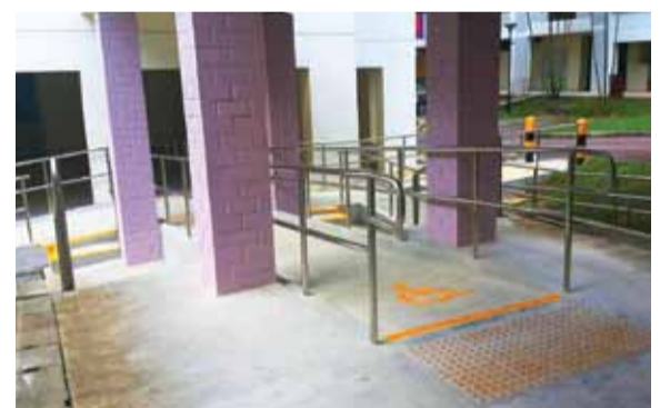
Barrier free access between Blk 623 and 628A Bukit Batok Central
