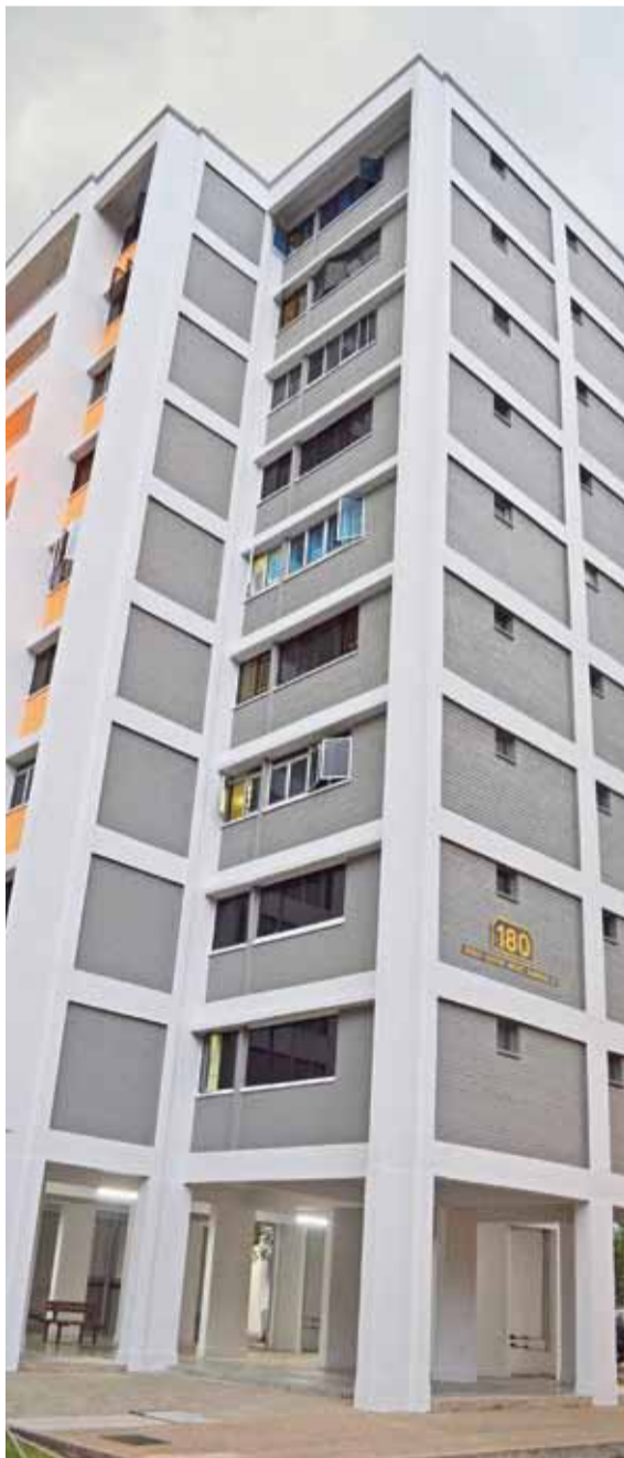
Repainting works for Blks 178 to 187 Bukit Batok West Ave 8
