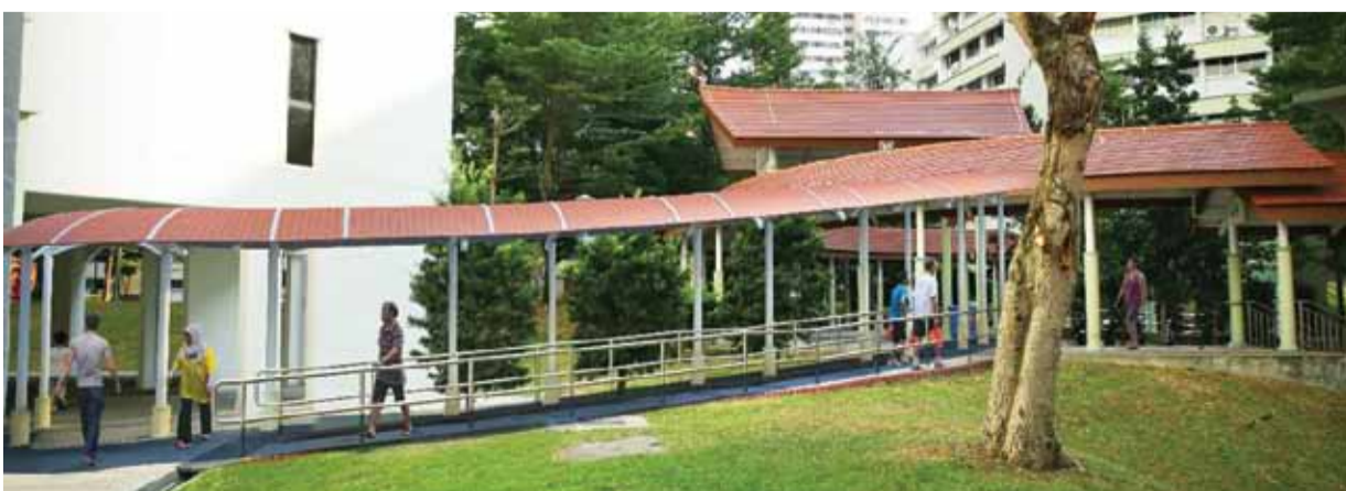
Covered linkway from Blk 110 Bukit Batok West Ave 6 (In Progress)
