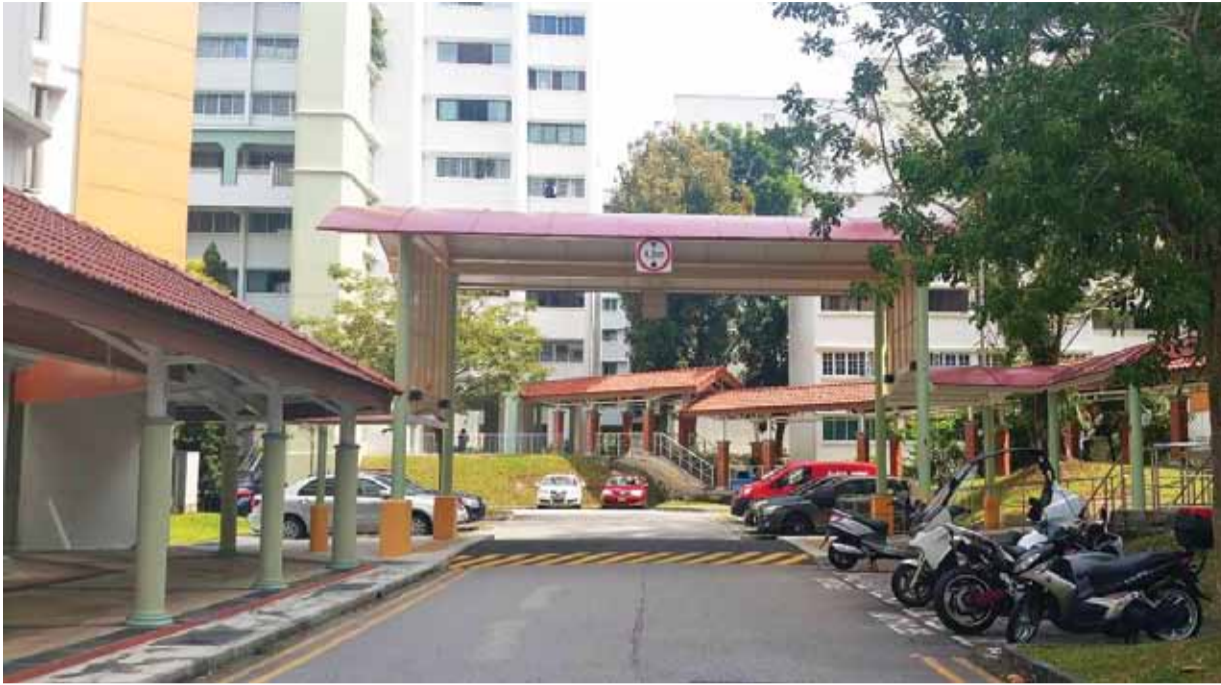
High and low covered linkway between Blk 103 and 106 Bukit Batok Central
