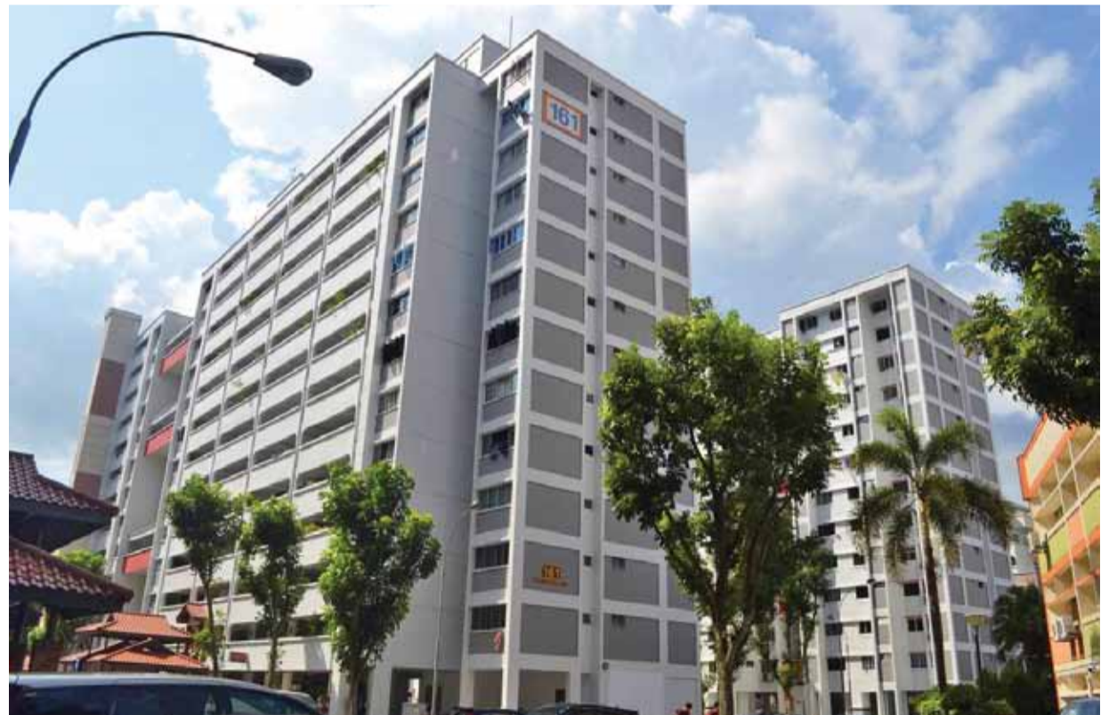
Repainting works at Blk 160 to 168 Bukit Batok West Ave 8
