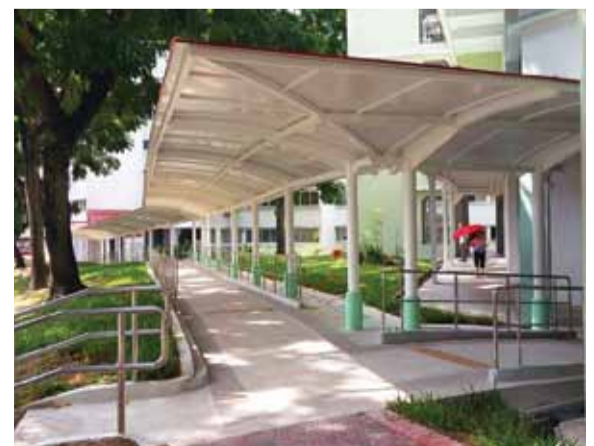
Covered linkway from Blk 103 to 104 Bukit Batok Central
