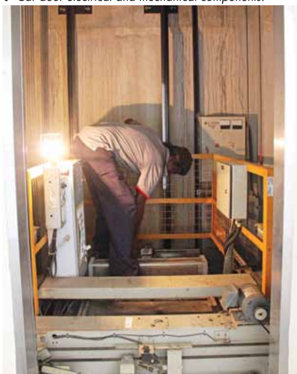
✓ Car top, car door operator, safety and limit switches.
