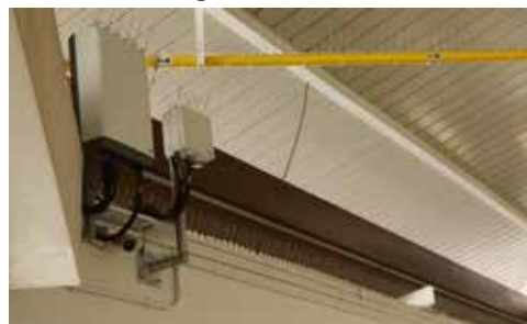
Installation of bird deterrent wire & netting
