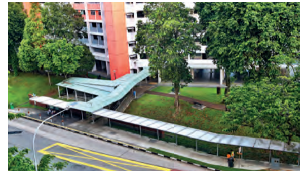
Covered linkway over BFA ramp at Block 335, Clementi Avenue 2.
