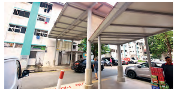
High linkway between Blocks 279 and 280, Bukit Batok East Avenue 3.
