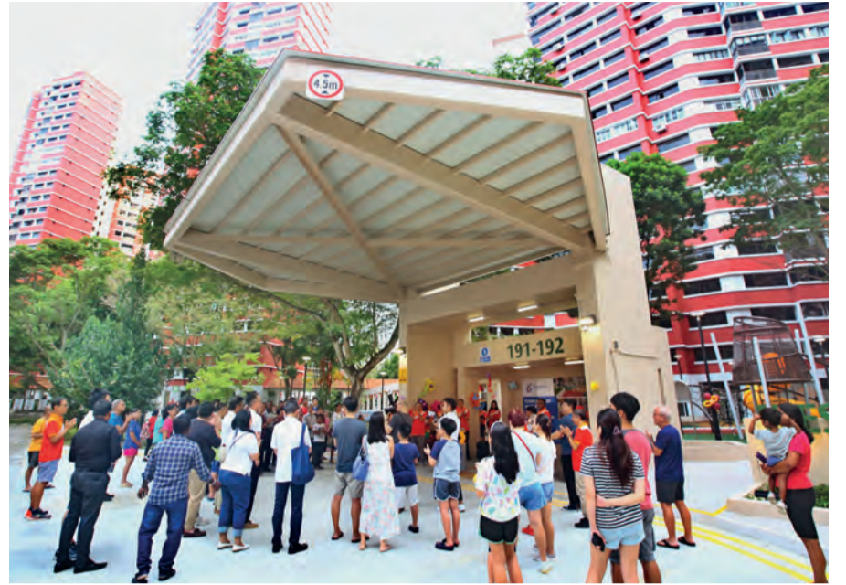
A new sheltered pavilion and drop-off point offer residents greater convenience.
